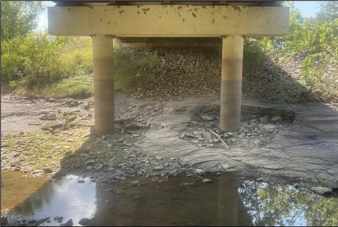
Bent # 3 footings are well keyed into solid shale.
