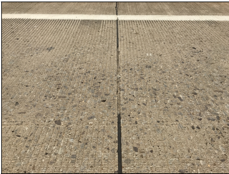
Span #2-Missing sealant in sawn deck joint.
