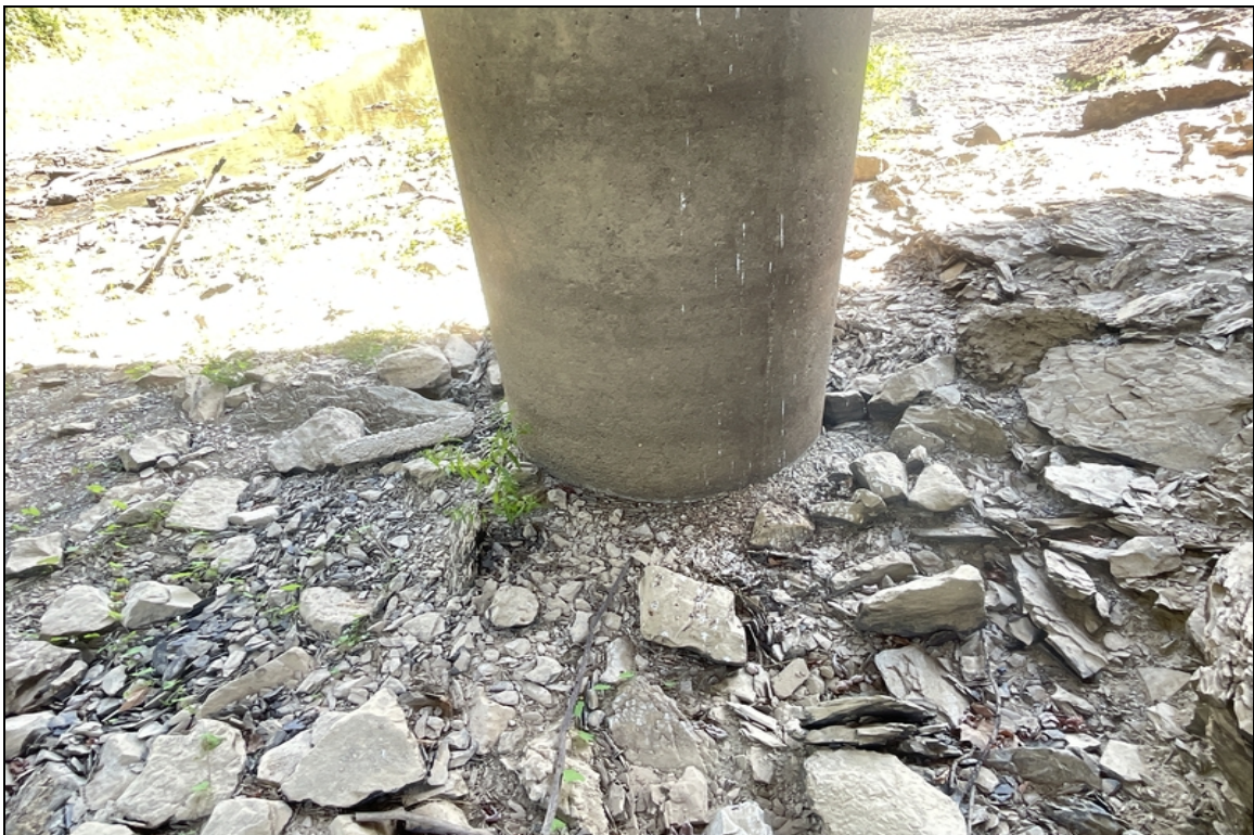
The base of Bent # 3 columns in the channel have light abrasion.
