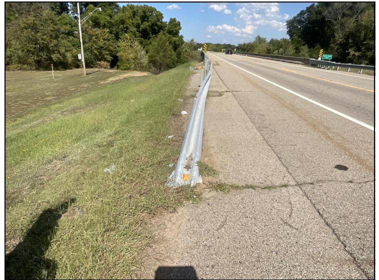
Minor collision damage to the Northwest approach guardrail.
