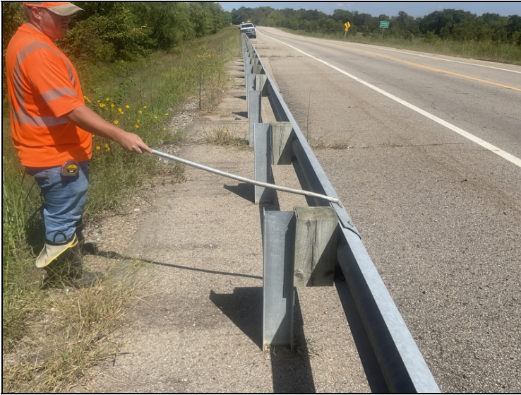
The Northeast approach guardrail is missing one timber spacer block and has a loose bolted connection.
