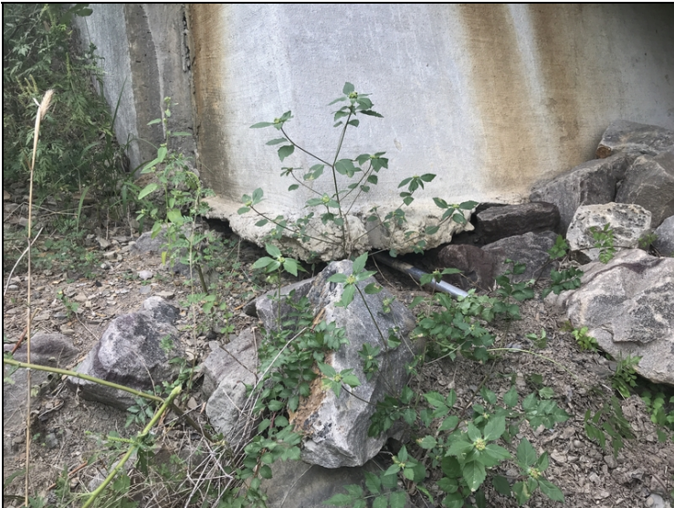
The right side of abutment #1 has minor earth settlement that has created a void approximately 2' long that penetrates the full width of the bridge seat.
