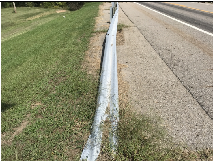
Abutment # 2 Rt approach guardrail damage.
