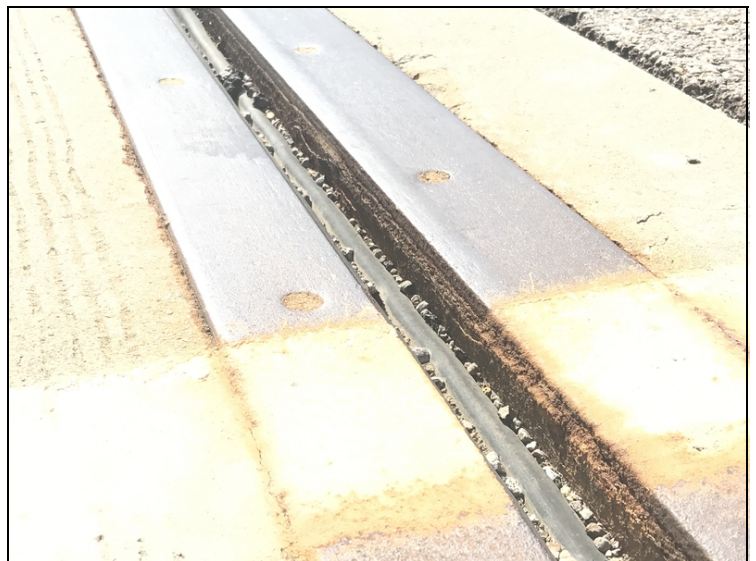
Abutment #2-Pack rust in expansion joint assembly.
