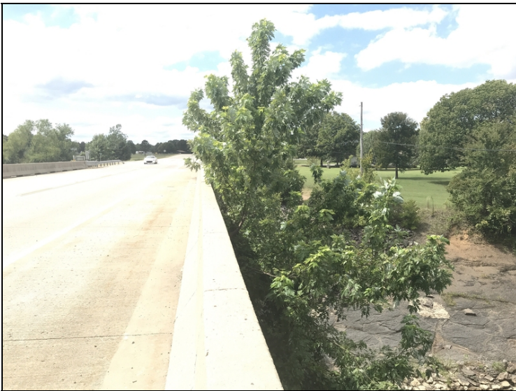
The channel has vegetation growing over the parapet on the North side of structure.
