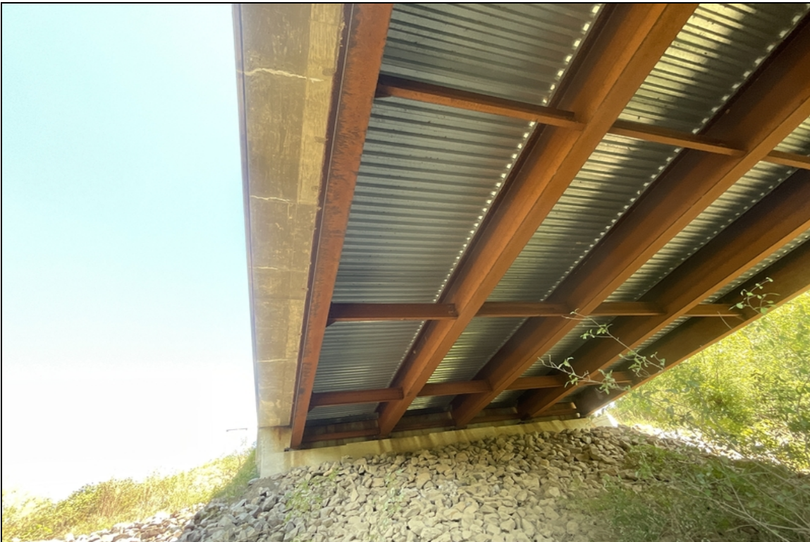
Deck soffit. Typical. Right overhang of Span # 1.
