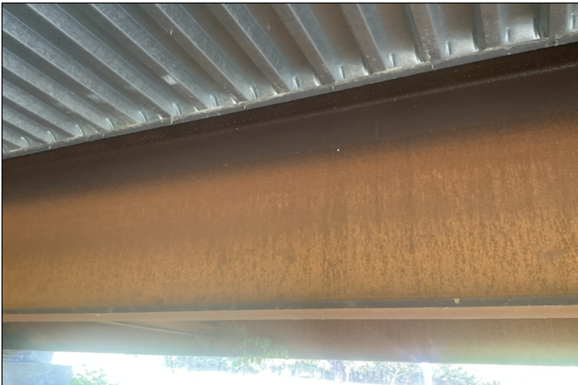
Steel protective coating. Superstructure. Typical.
