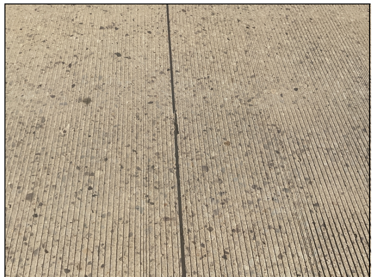
Deteriorated transverse saw joint sealant.
