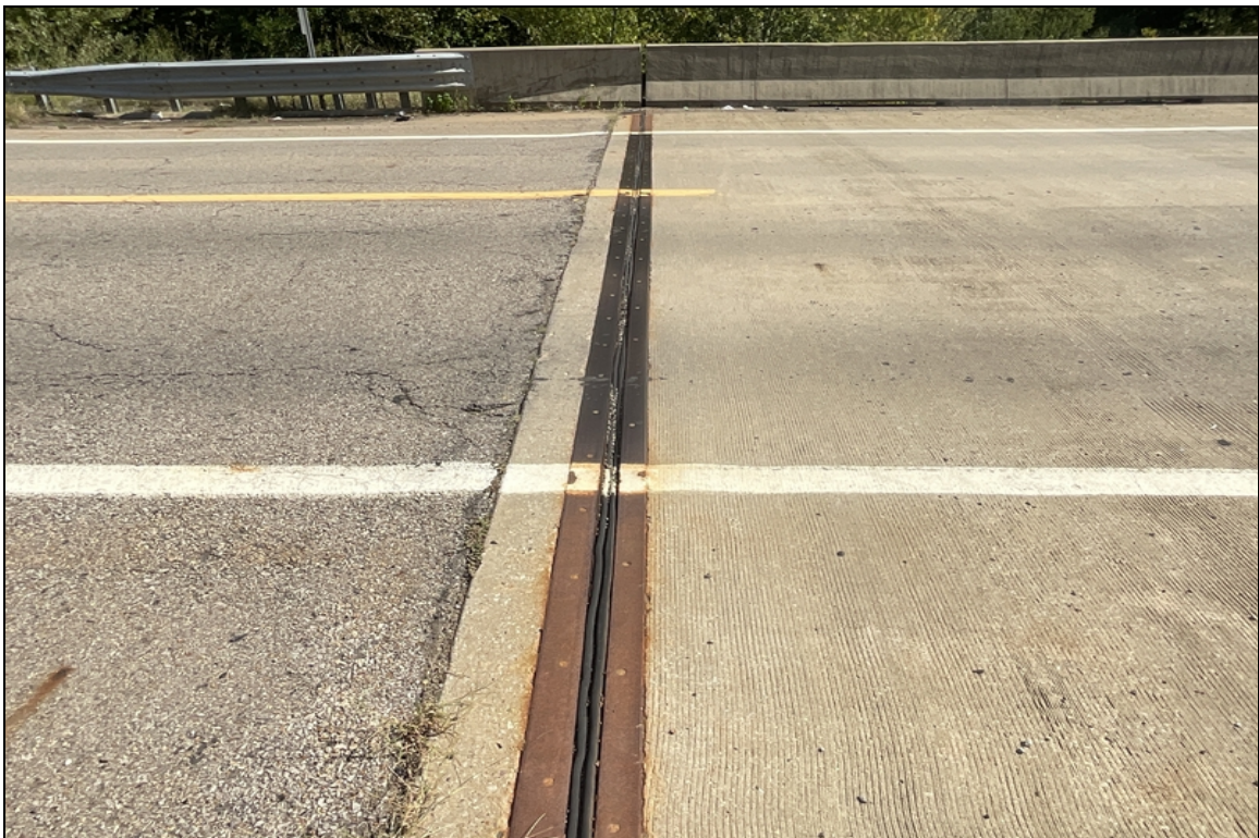
East abutment expansion joint seal.
