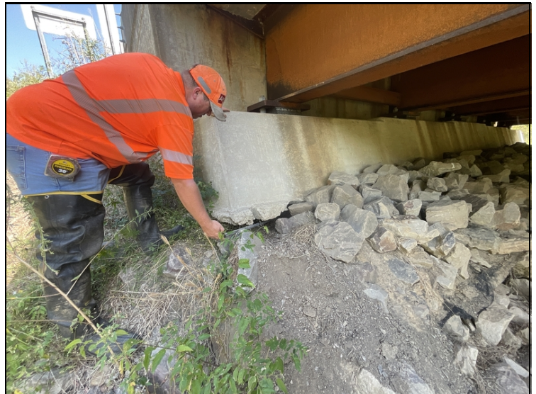
Minor earth settlement under the Right side of Bent # 1.
