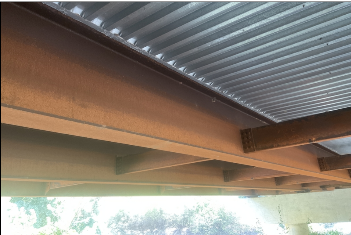
Abnormal weathering (Reddish color) of the protective steel coating.
