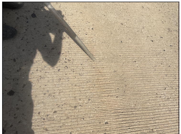
Deck. Sealable Longitudinal crack.
