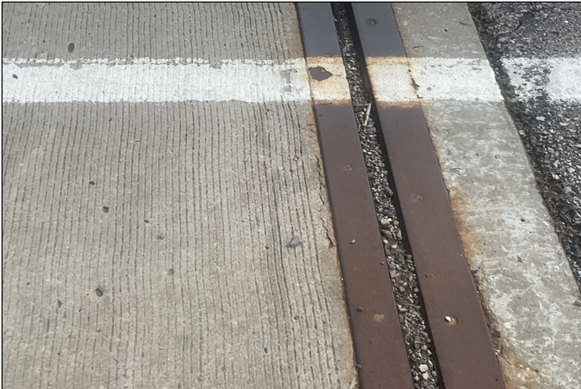
Minor delaminated areas and spalls in the deck adjacent to the expansion joint at the West abutment.
