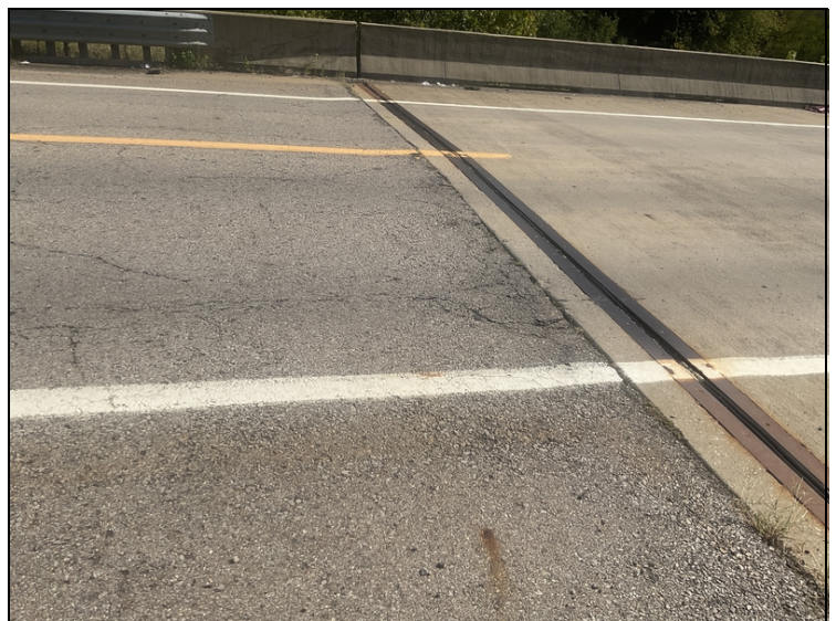
Approach roadway at the East abutment. Asphalt settlement.
