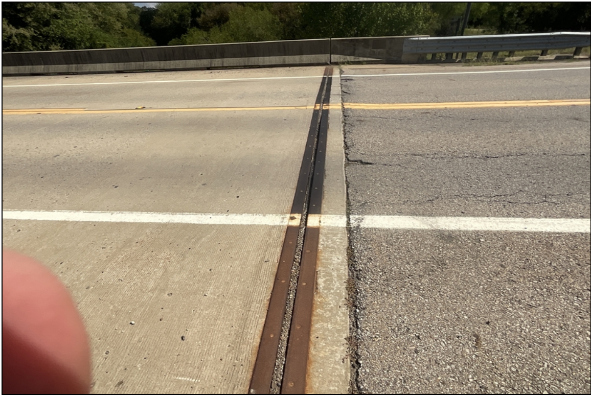
Expansion joint seal at the West abutment.
