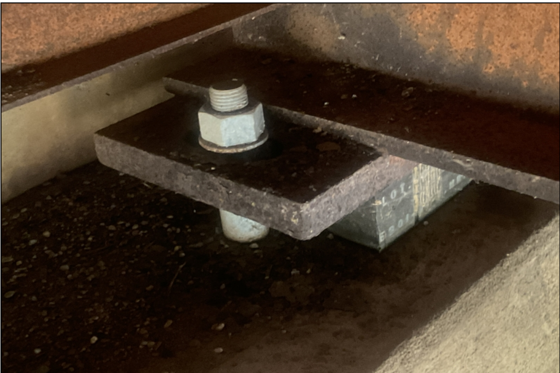
Beam # 4. Bent # 4. Minor corrosion with flaking rust.
