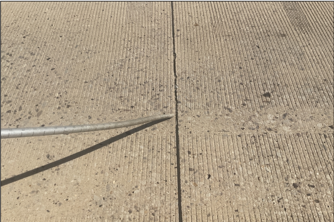
Deteriorated transverse saw joint sealant.
