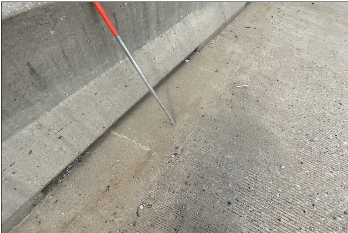
Transverse cracks in the right gutter.
