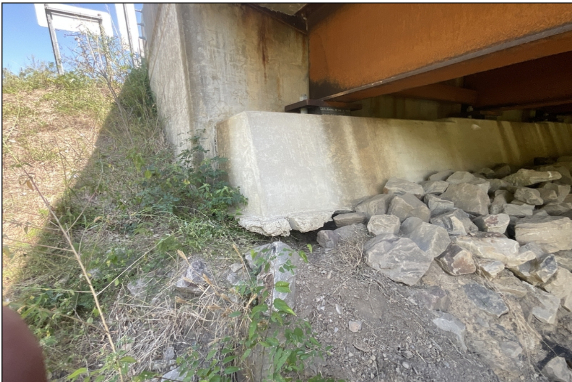
Minor earth settlement under the right side of Bent # 1.
