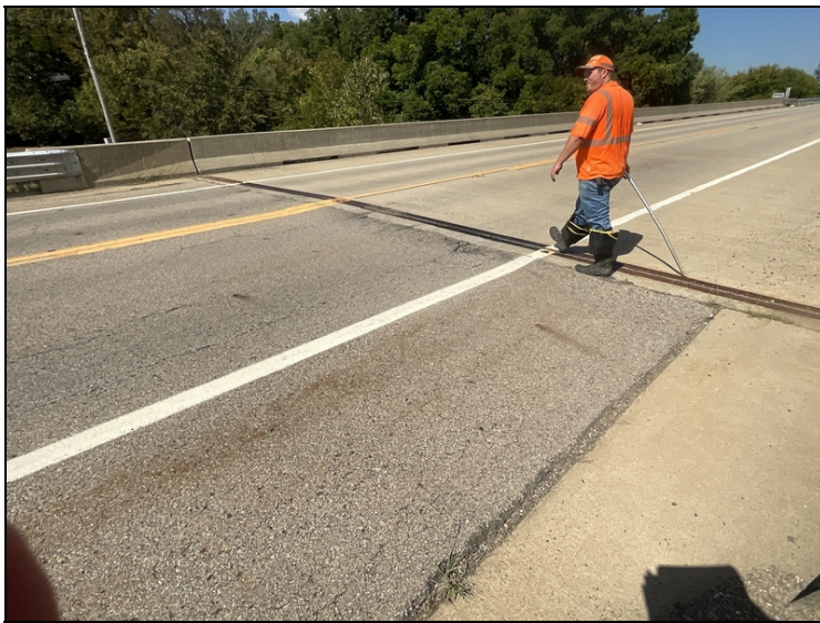
Approach roadway at the West bridge end. Asphalt settlement.
