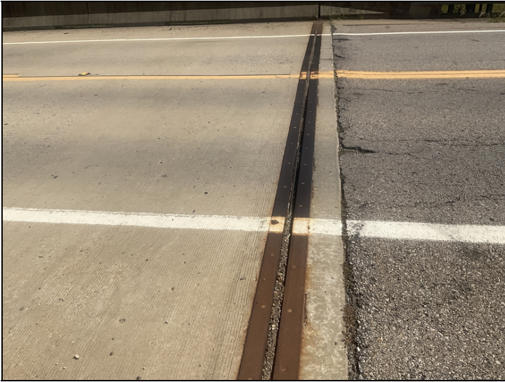
West abutment. Settlement of the expansion joint seal.
