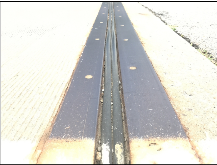
Abutment #1 compression joint seal-Adhesion failure.
