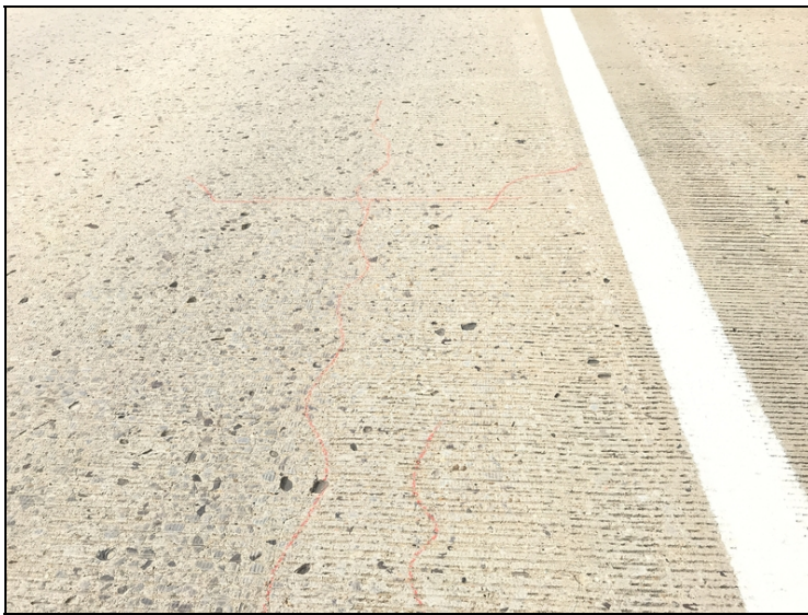
Span #1-Longitudinal and transverse deck cracking.
