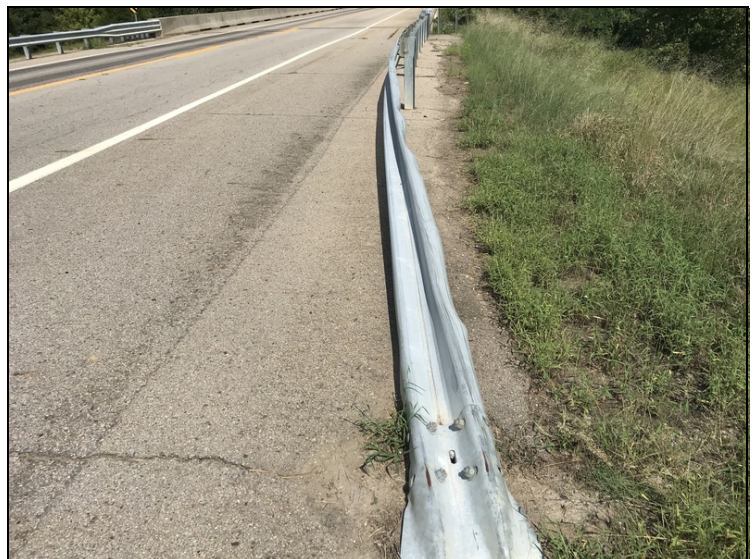
Abutment # 2 Lt approach guardrail damage.
